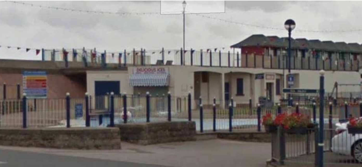
A recent image (above) shows the colonnade with beach huts above. This shows the Ice Cream Kiosk, seen in the RIBA photo, but now with infill to its left and right, and some of the arcades of the colonnade prior to being temporarily infilled with plywood following structural report recommendations in 2018. Since this time, the remaining arcades have also been blocked with plywood for the same reason.
