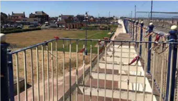
Photo taken from south end of promenade, on top of the colonnade (original 1930’s section) looking north over the gardens. The structural plan of the garden has not changed since constructed in 1953. The bowling green is seen in the middle of the photo, beyond is the flower garden, and beyond that, the tennis court. Note the ribbons on the railings, a symbol of the feelings of the local community about the loss of the beach huts and colonnade.
